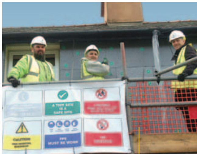
Cavity wall insulations are a key part of Energy Services' work
