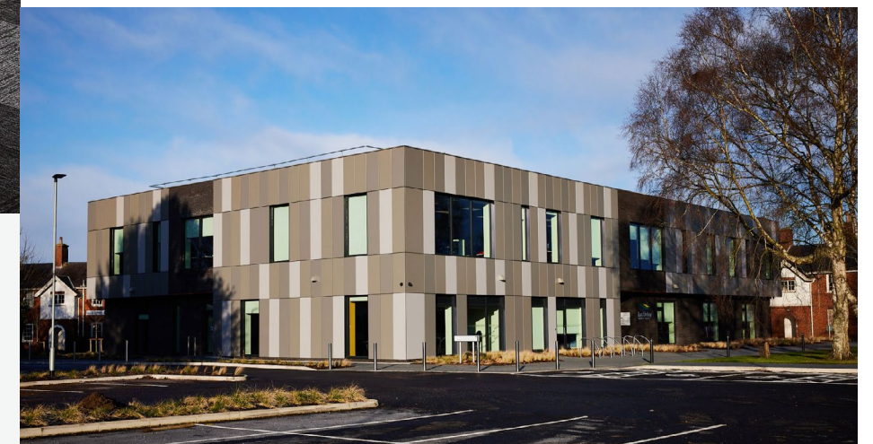
Taking a fabric-first approach to the Public Sector Hub allowed us to achieve high levels of insulation, making the building more energy efficient
