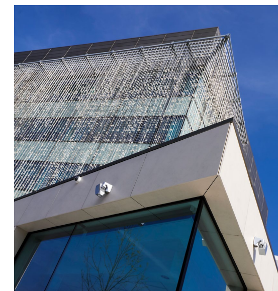
The fibre optic lights on the BioCity Discovery Building also provide solar shading to reduce heat gain through the large glass windows
