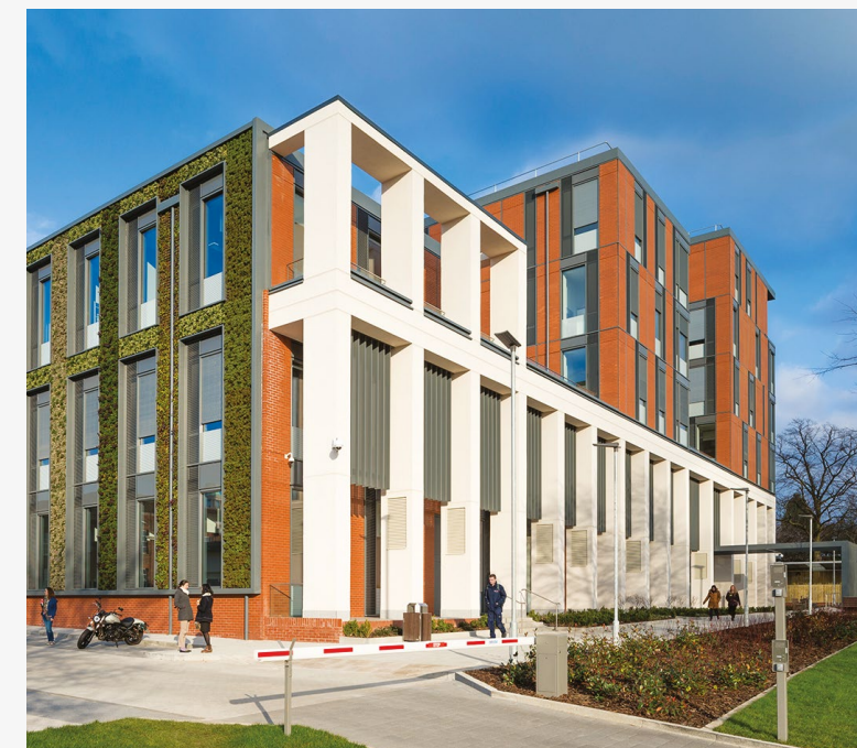
Left: The George Davies Centre of Medicine at the University of Leicester, completed by Willmott Dixon in 2016.
