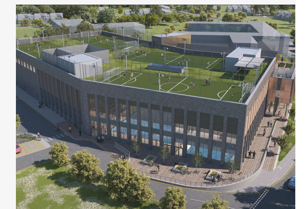
Below: Spelthorne Leisure Centre in Surrey, which is currently under construction.
